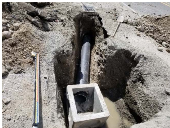
Surface Water Structure Repair
